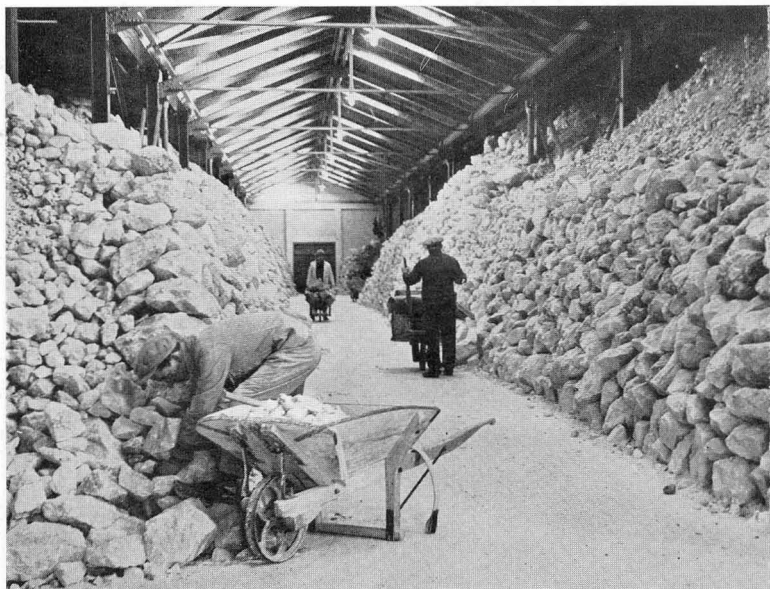
FIG. 13. Raw cryolite store. Transporting material by wheelbarrow.
