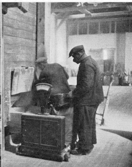
FIG. 15. (a) Hand-sorting larger pieces of cryolite. (b) Packing the finished product in sacks with a shovel.
